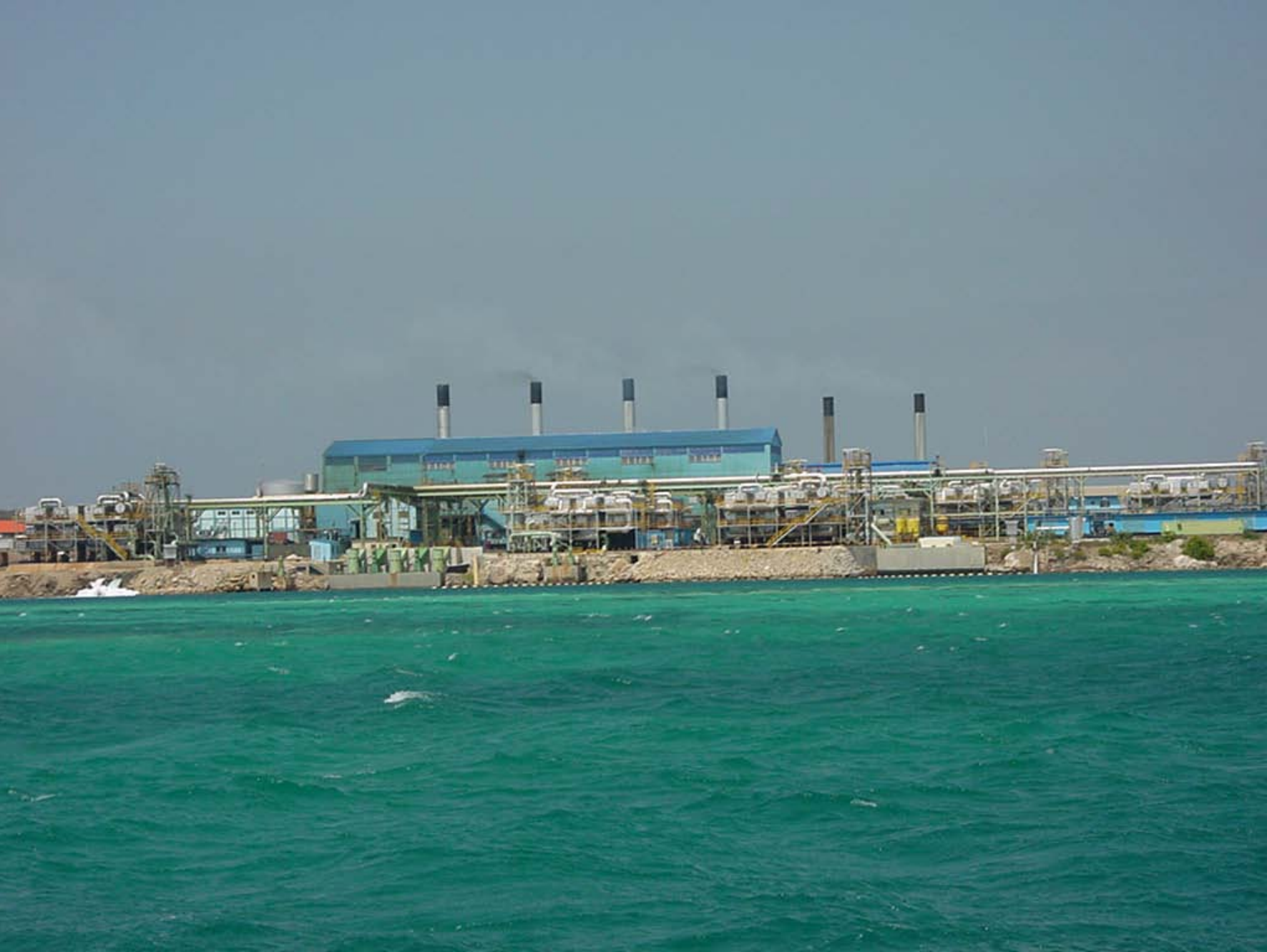
Desalinization plant on southwest coast near DePalm Island
